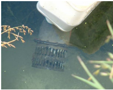
Figure 48. Check water inlets are clean and free of obstructions.
