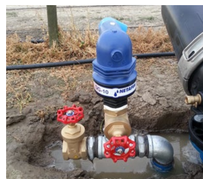
Figure 23. Air relief valve.
