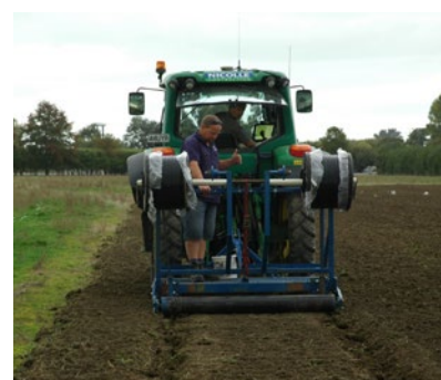
Figure 30. Laying buried dripline: RTK-GPS guided tractor, roller for depth control.
