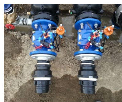
Figure 22. Solenoid valve take-offs.
