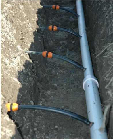
Figure 17. Buried PVC header for sub-surface drip.
