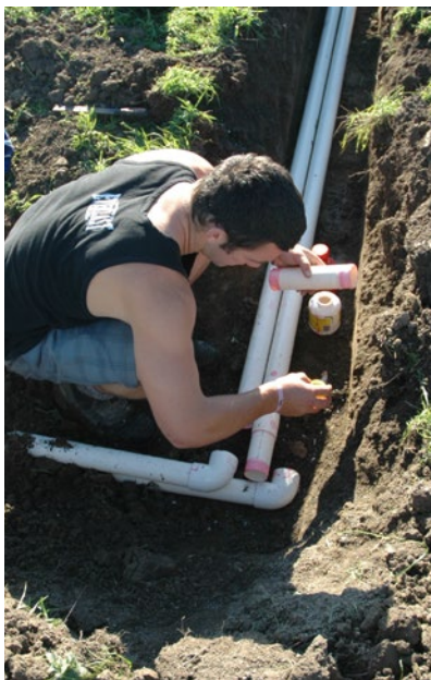
Figure 32. Ensure all joints are correctly made and water tight.
