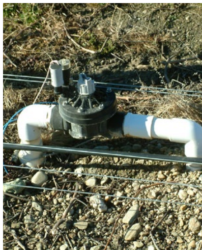
Figure 24. Solenoid valve allows automatic block switching.
