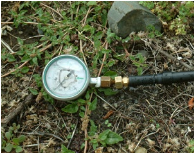
Figure 41. Checking pressure at the end of a dripline.
