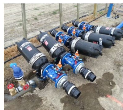
Figure 21. Semipermanent headworks with filters, solenoid valve take-offs and air relief.
