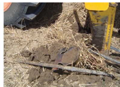
Figure 55. Lifting buried dripline prior to recovery for re-use.
