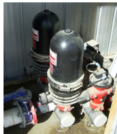
Figure 20. Twin filters set up to enable automatic back flushing. Filtered water from one filter flows back through the other to ensure proper cleaning.
