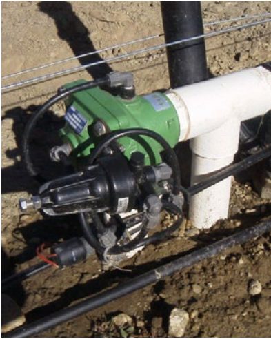
Figure 12. Pressure regulators ensure pressure does not exceed maximum allowed.
