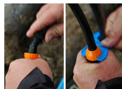
Figure 39. Joining dripline mid-row (left). Joint to be pulled into soil by machine. Ensure all connections are secure. Once buried they are difficult to check and repair.
