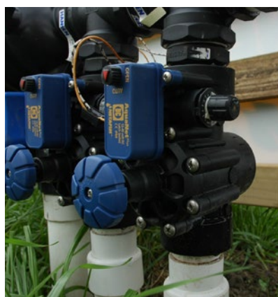
Figure 26. Electric solenoid valve with in-built adjustable pressure regulator and manual close.
