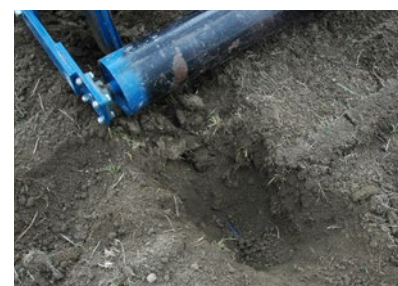
Figure 37. Installation depth should be checked regularly. On this machine, the back roller controls the depth.
