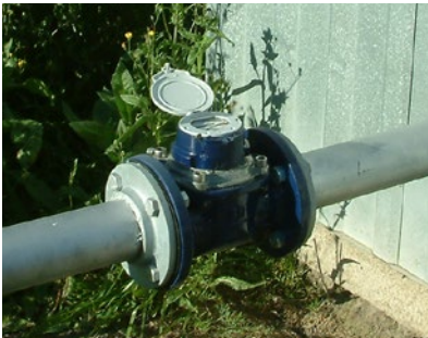
Figure 42. Check flow rates, block by block, are as specified in the design.
