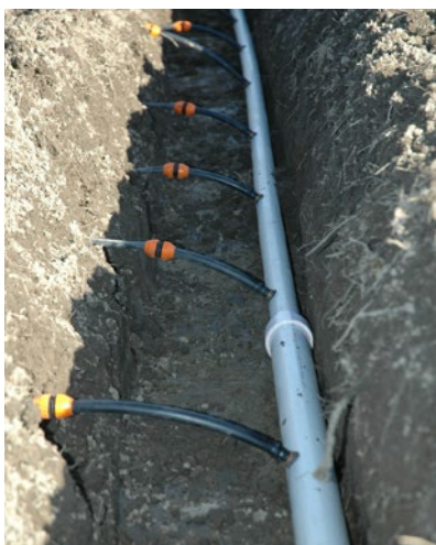
Figure 33. PVC sub-main (header) with off-takes connected to buried driplines.
