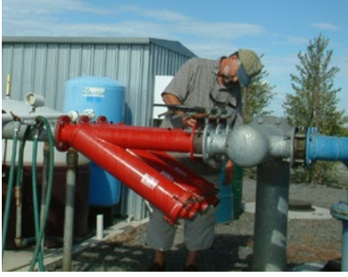
Figure 40. Checking system pressure at the headworks of a larger drip irrigation system.
