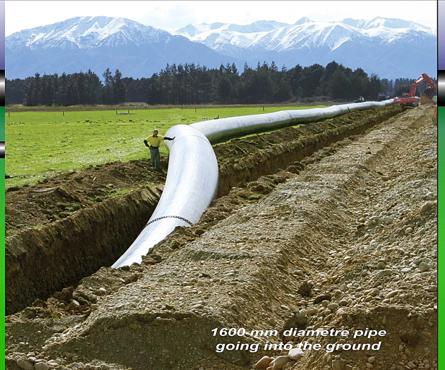
Large Bore PE Pipe factory in the field
